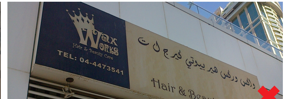
This sign is unacceptable it is faded dirty with exposed wiring.
