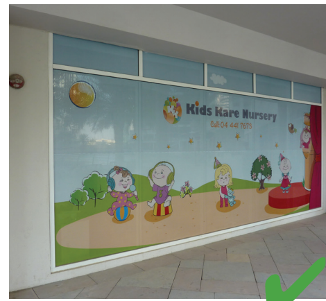
A children's nursery with appropriate vinyl obscuring the windows and adding privacy and shade.
